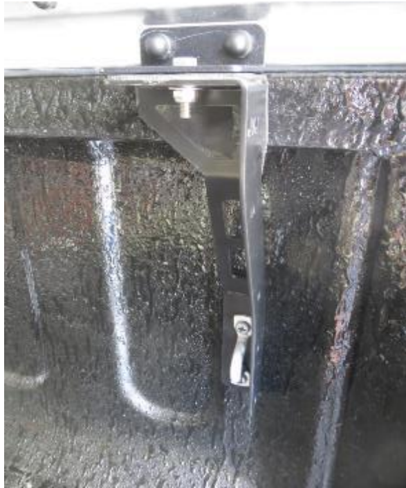
Figure 18: Rear-Right Support Bracket Installed
